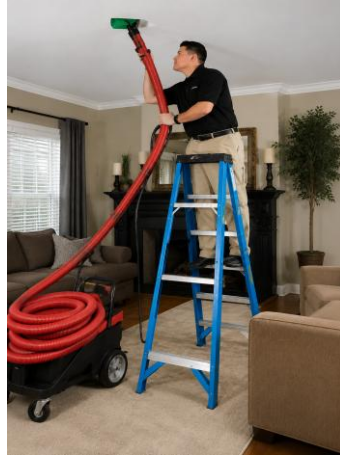
Air Duct Cleaning
